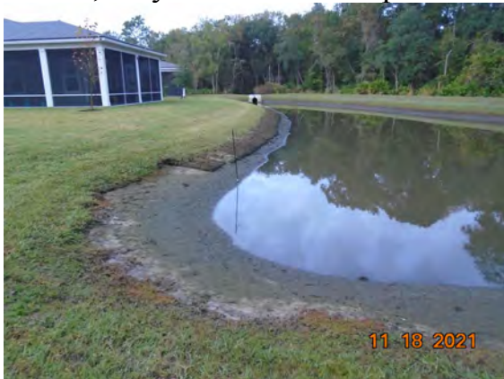
Pond 4: Had complaint for grasses growing around pond. No vegetation noticed, only where sod was placed too low on new construction.
