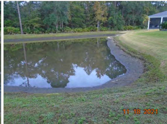
Pond 4: Had complaint for grasses growing around pond. No vegetation noticed, only where sod was placed too low on new construction.
