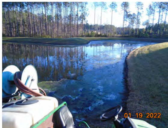
Pond 2: Vegetation decaying around pond.
