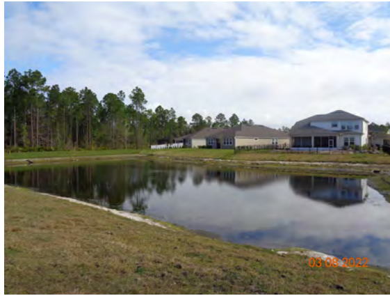
Pond NN: Perimeter grasses are decaying.
