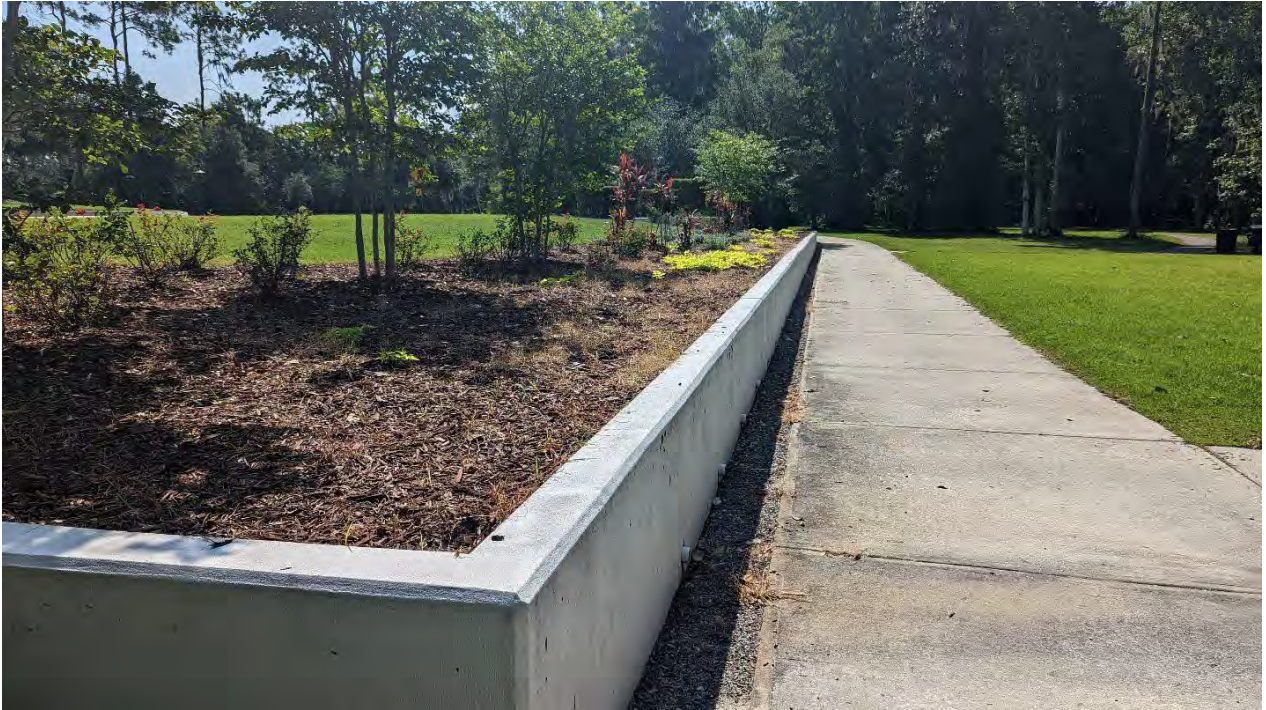
White Wall bed, missing vegetation
