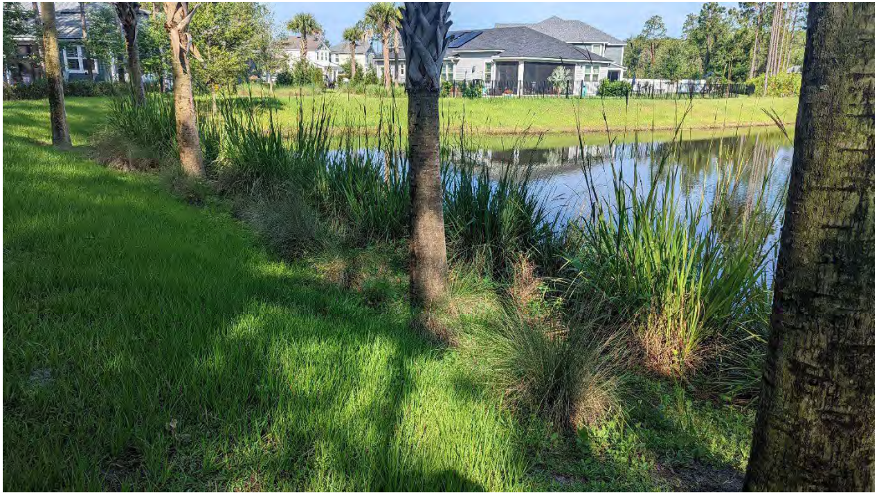
Pond AA at the end of Cloverbrook Rd., Pond banks not maintained
