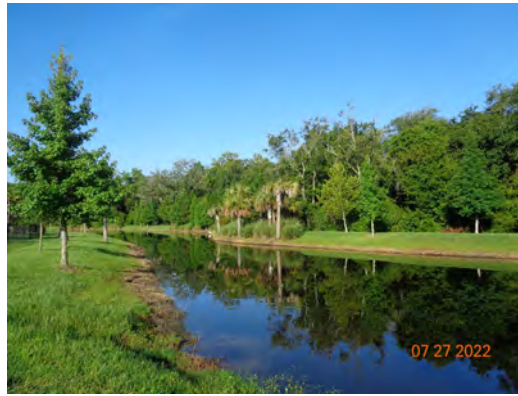
Pond T: Pond is in good condition.
