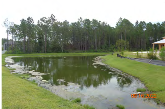
Pond GG: Pond in good condition, treated for algae and emergent weeds.
