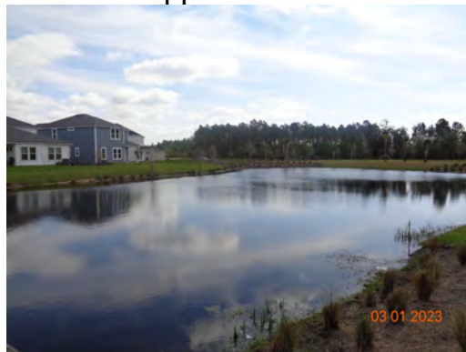
Pond II: Pond in good condition, algae noticed.
