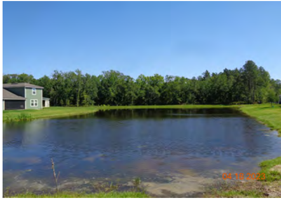
Pond AAA: Pond in good condition. Water level is low.
