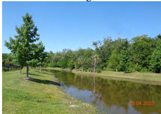
Pond T: Pond is in good condition.
