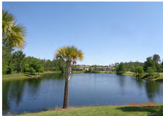
Pond S: Pond in good condition. No algae noticed.
