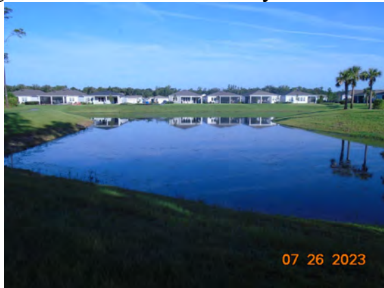
Pond 13: Vegetation is decaying.
