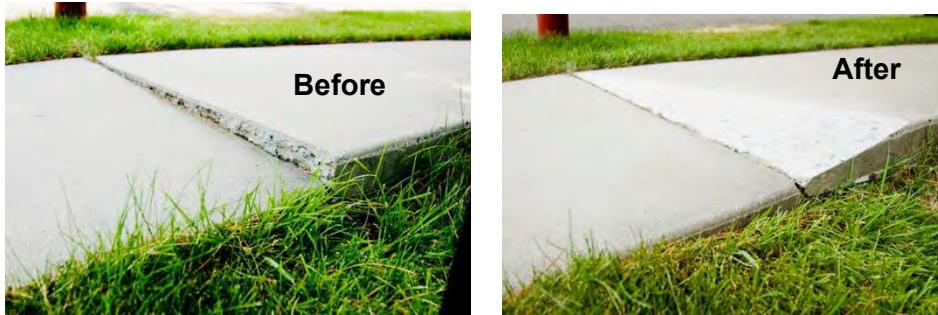
Figure 11: Precision Sidewalk Safety Work Example
